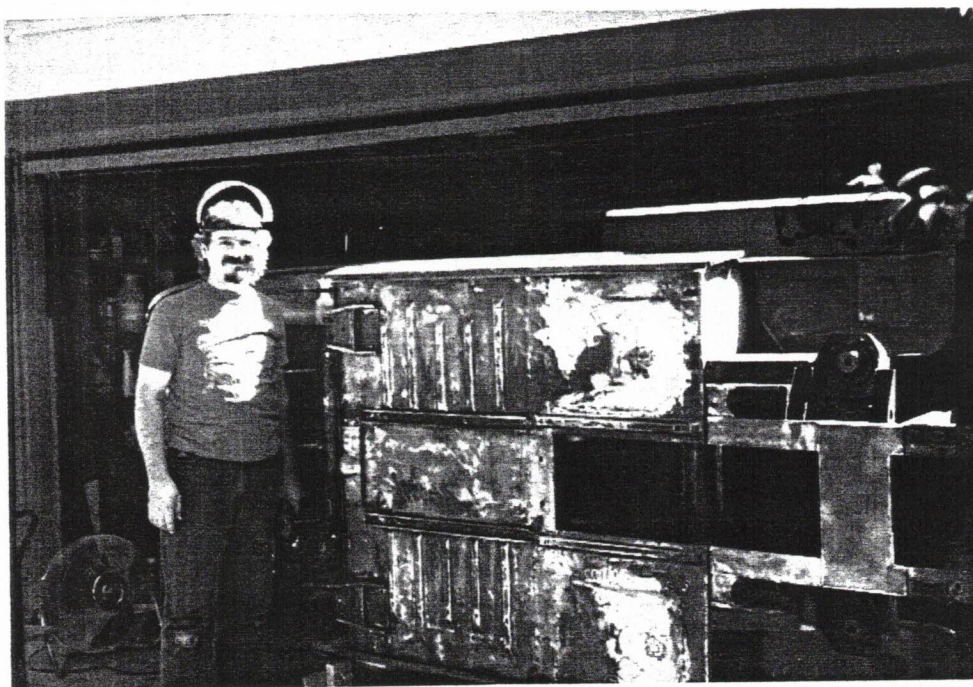
Here I am on my roll over jig so Craig could clean and repair some rust in preparation for painting. Craig cleaned down to metal before painting with rust resistant paint.
